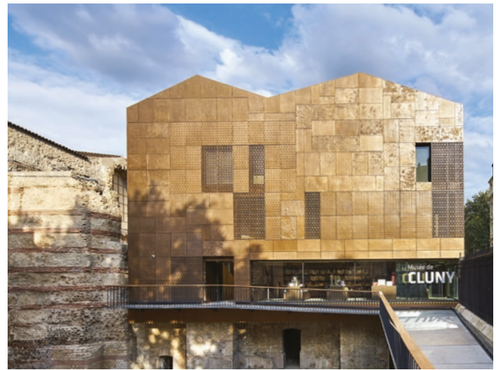
The Musée de Cluny—National Museum of the Middle Ages. View of the visitor reception building designed by Bernard Desmoulin (architect) in 2018, and the Gallo-Roman baths (1 st –2 nd centuries)
